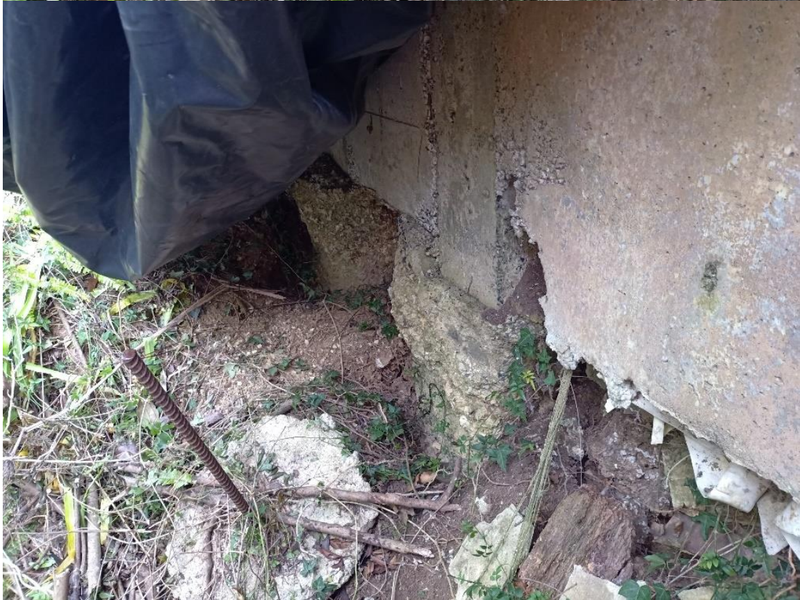
Photo 7: Exposed pile #2 & 3 showing scarp
