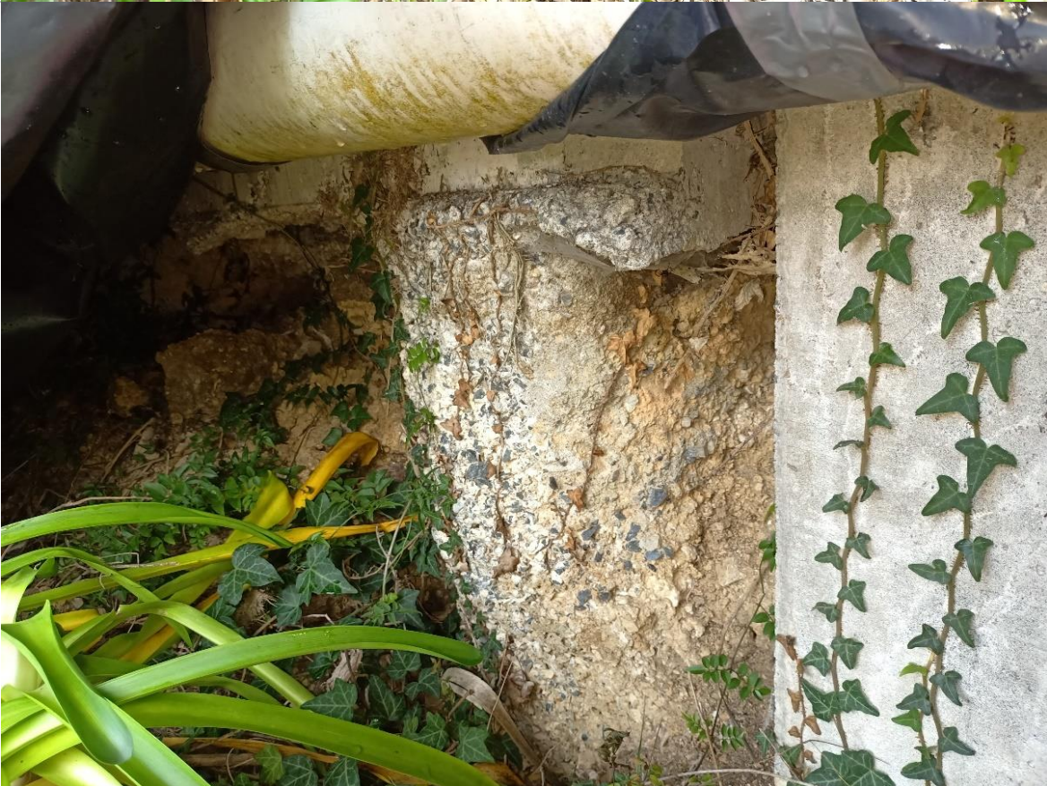
Photo 5: Western end where ground level is at concrete beam level
